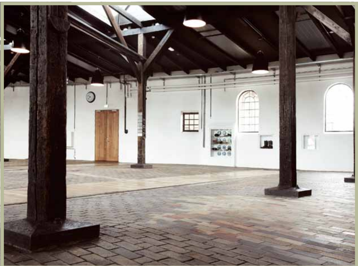
After the renovation
