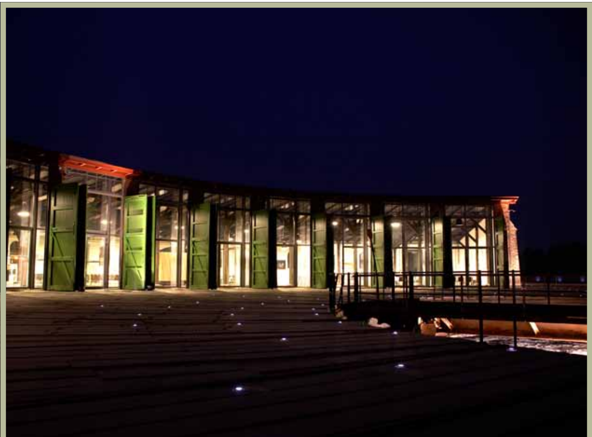
After the renovation
