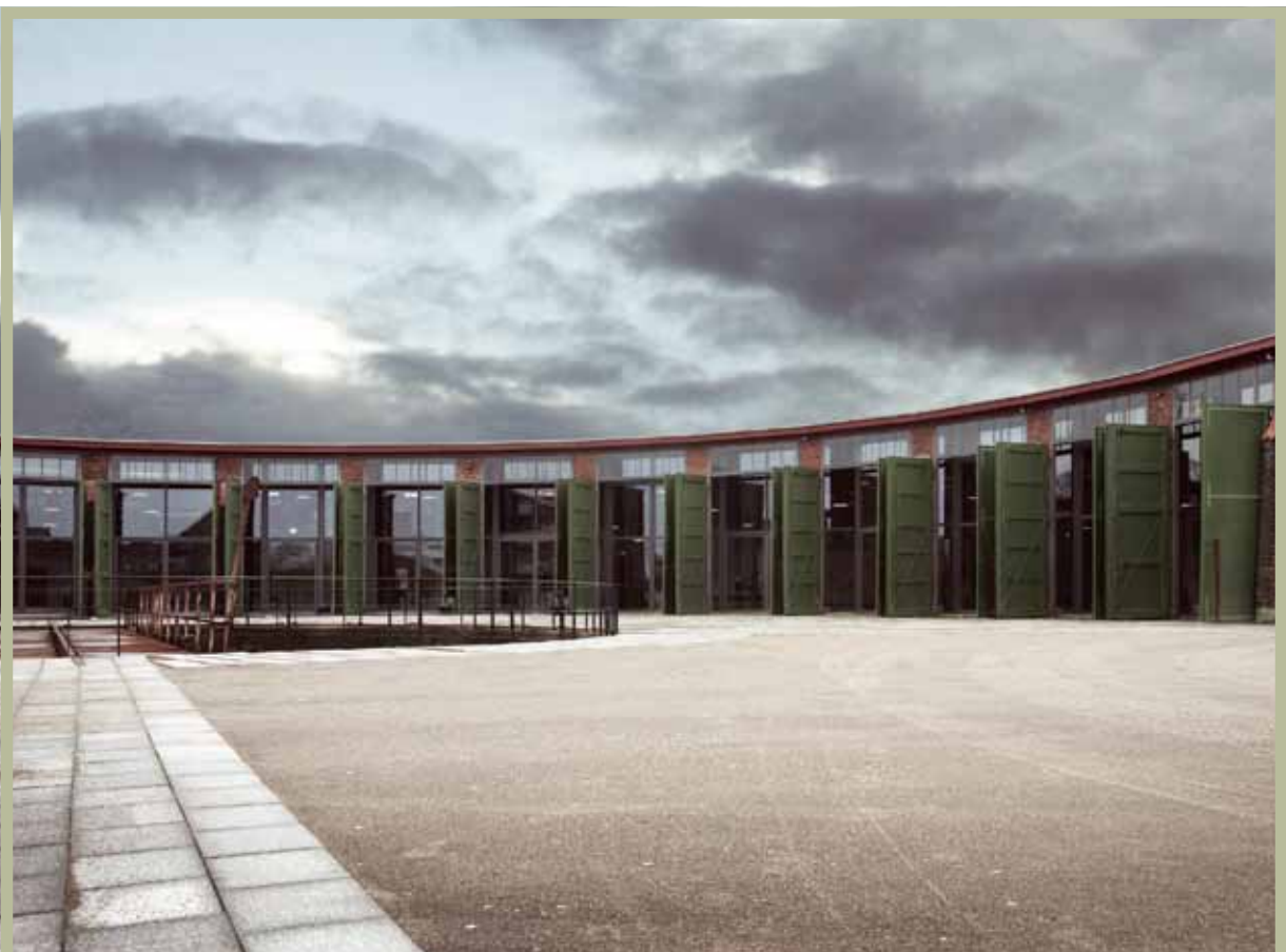
After the renovation
