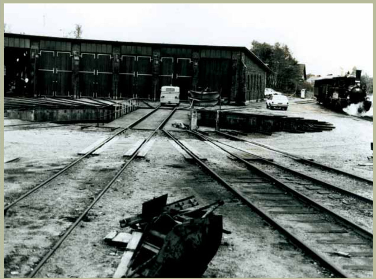
Before the renovation
