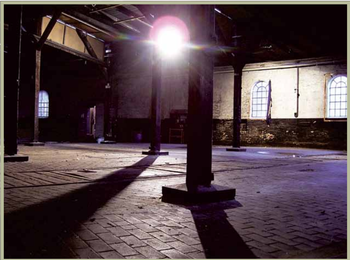
Before the renovation
