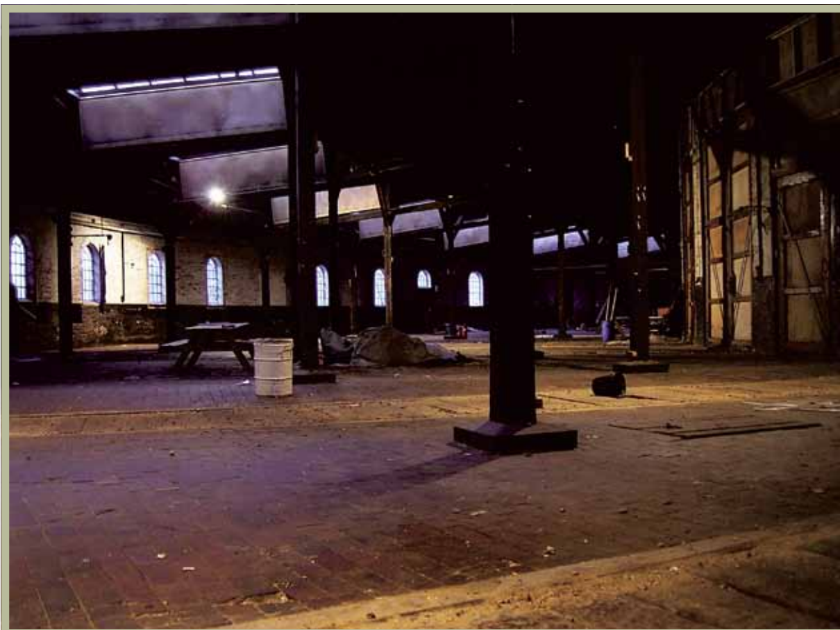
Before the renovation
