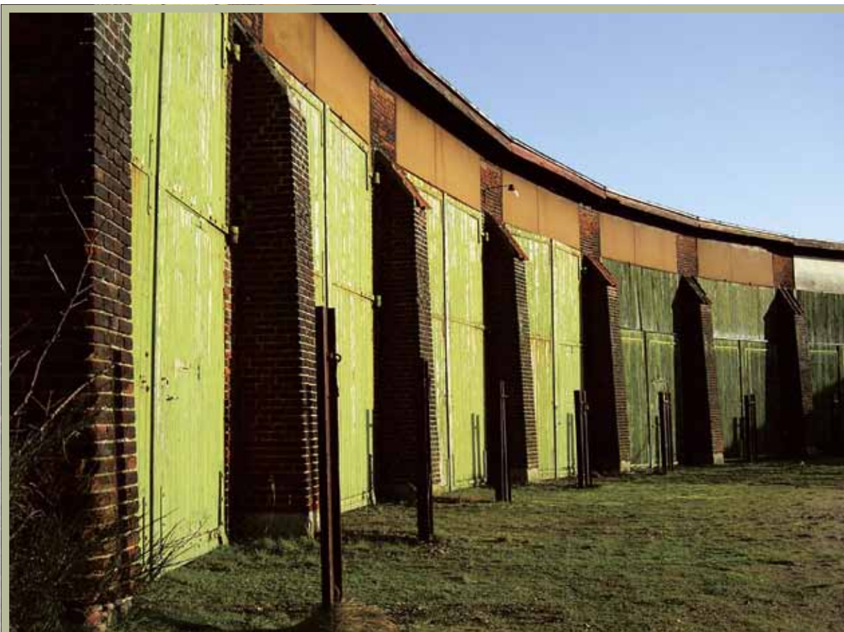
Before the renovation
