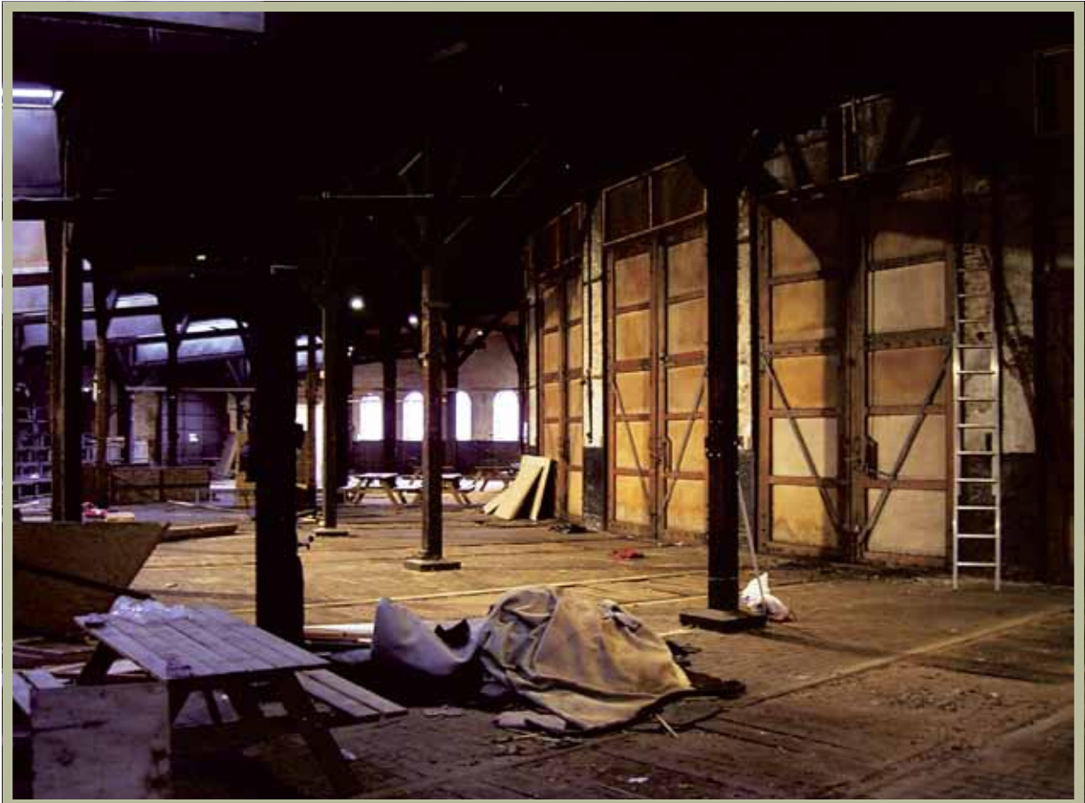
Before the renovation
