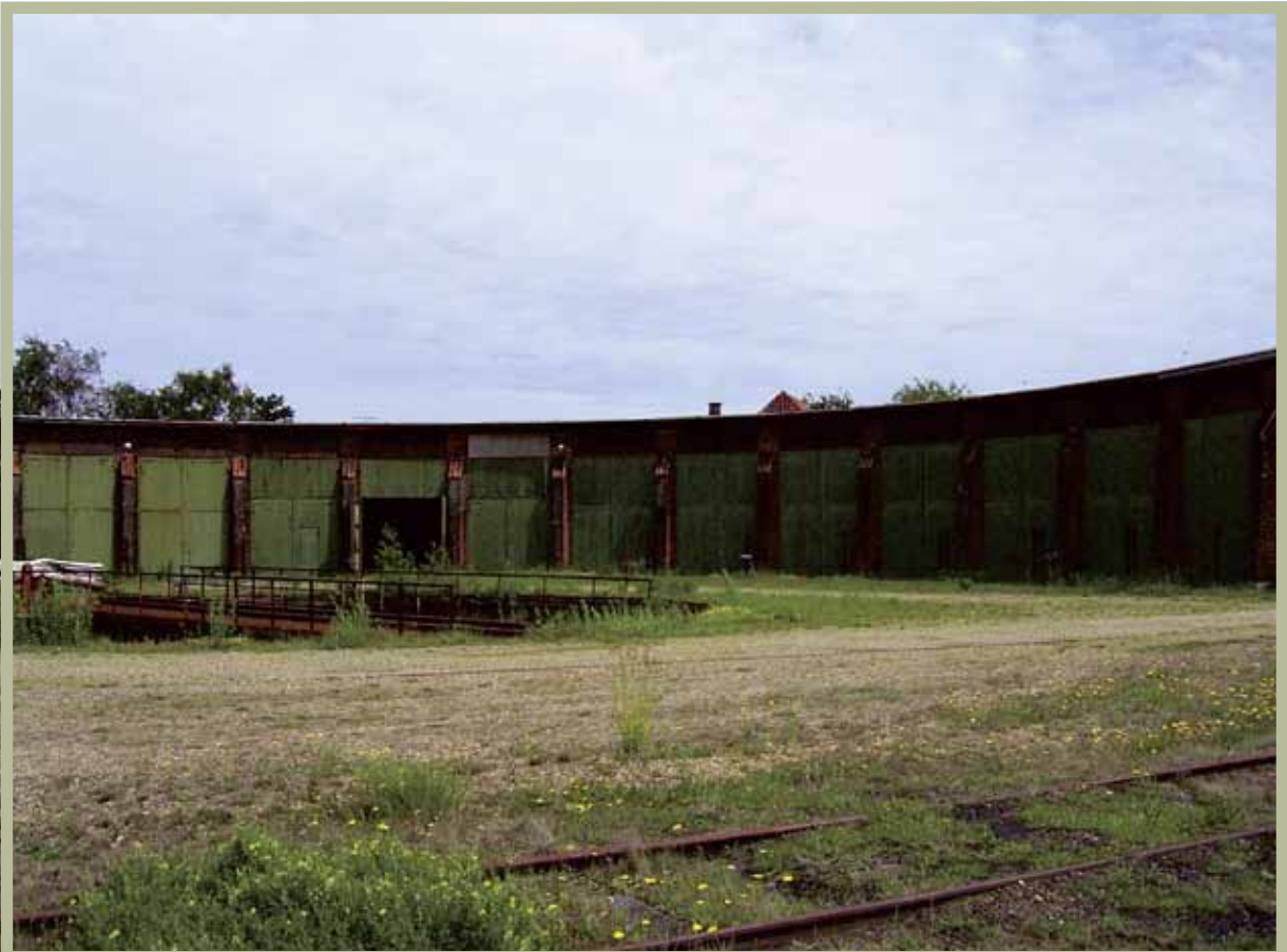
Before the renovation
