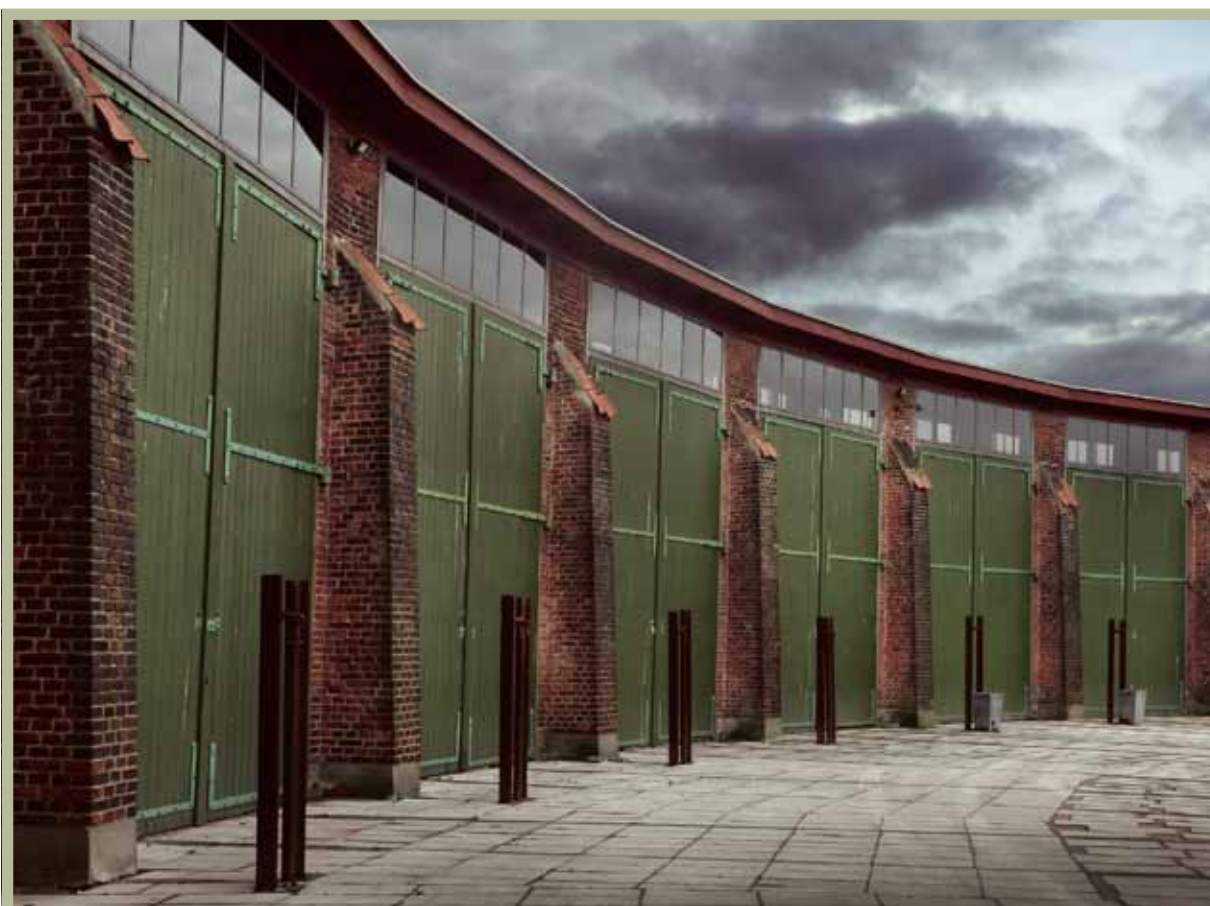
After the renovation
